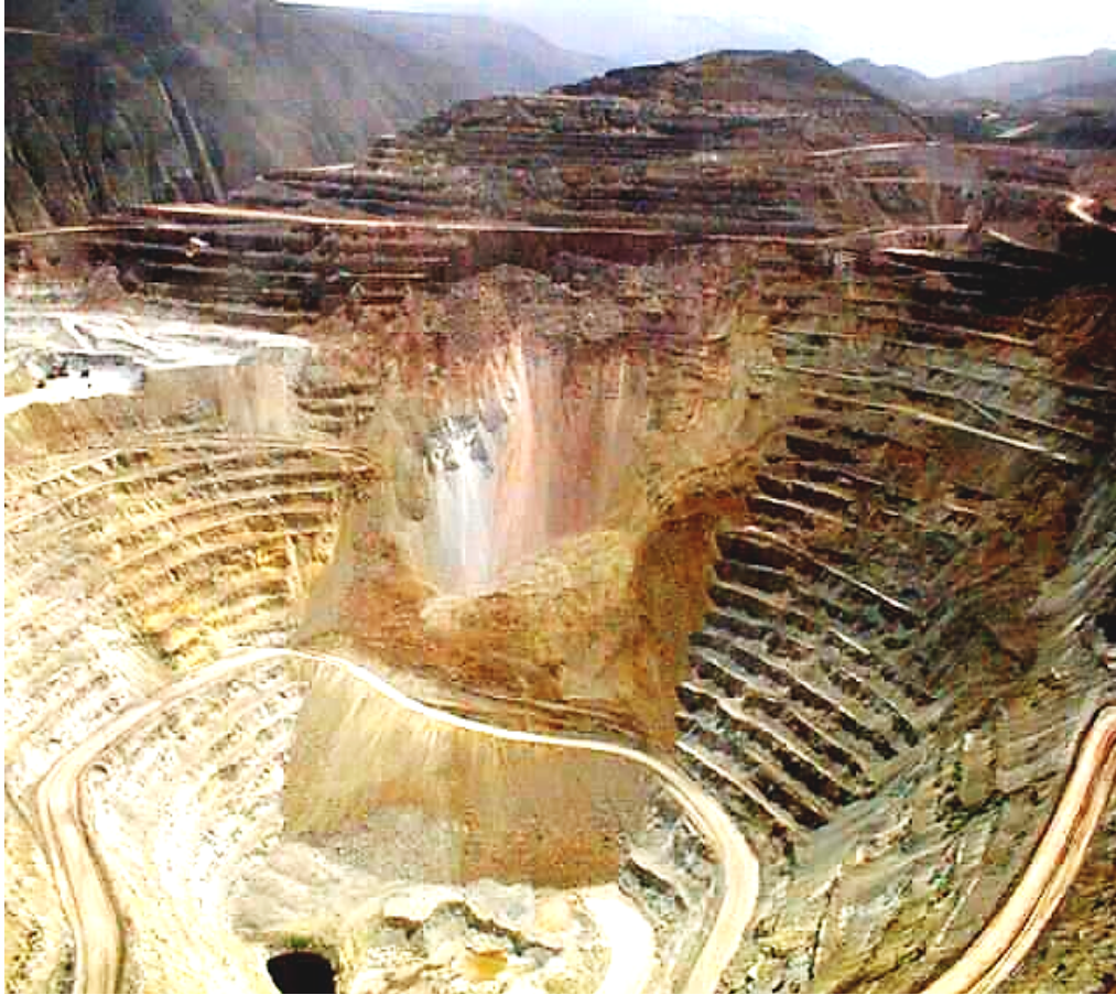
Figure 2: A large scale slope failure in an open pit mine.
