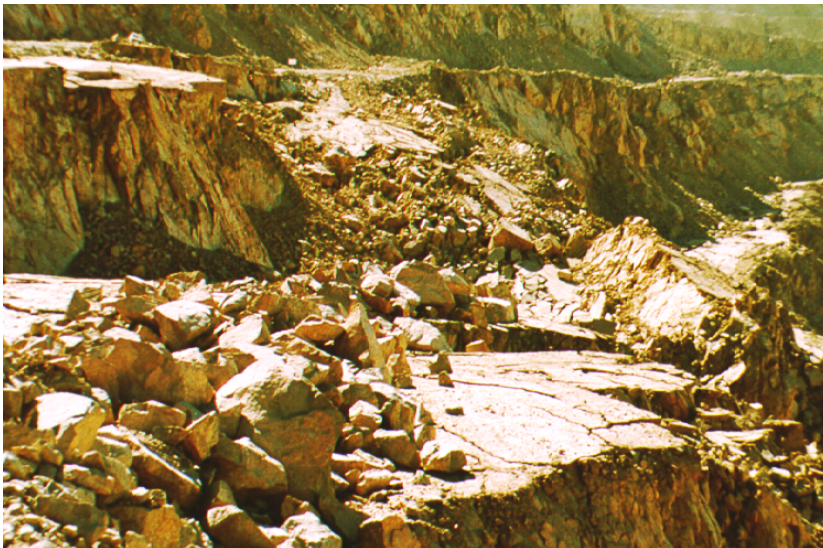
Figure 11: Large rock mass deformations in the West wall of the Chuquicamata Open Pit Mine in Chile.
