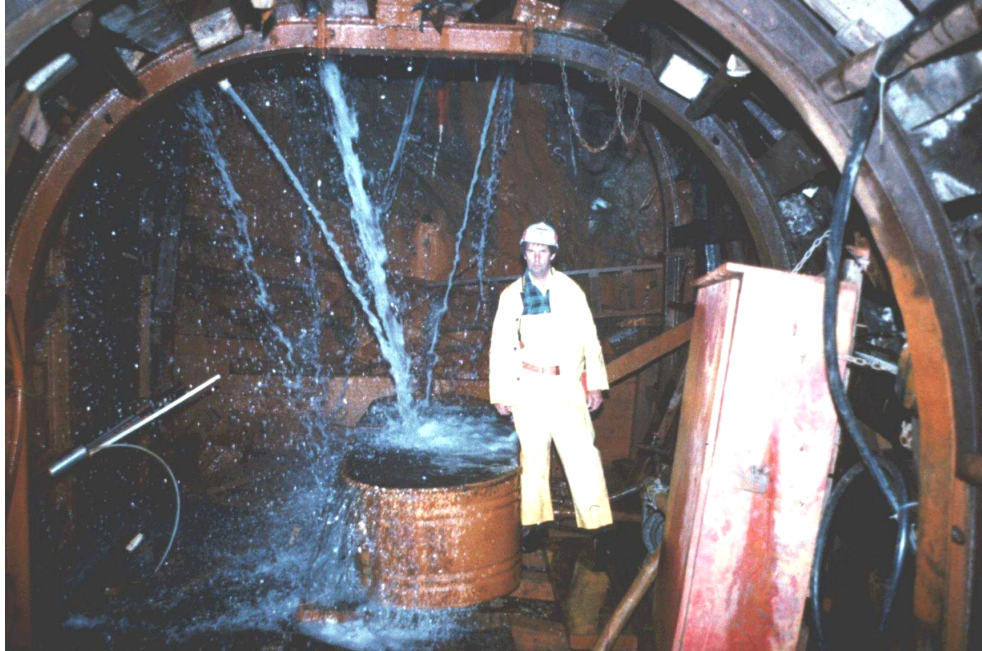
Figure 8: Collection of water from the boreholes drilled from the Downie Slide drainage gallery.
