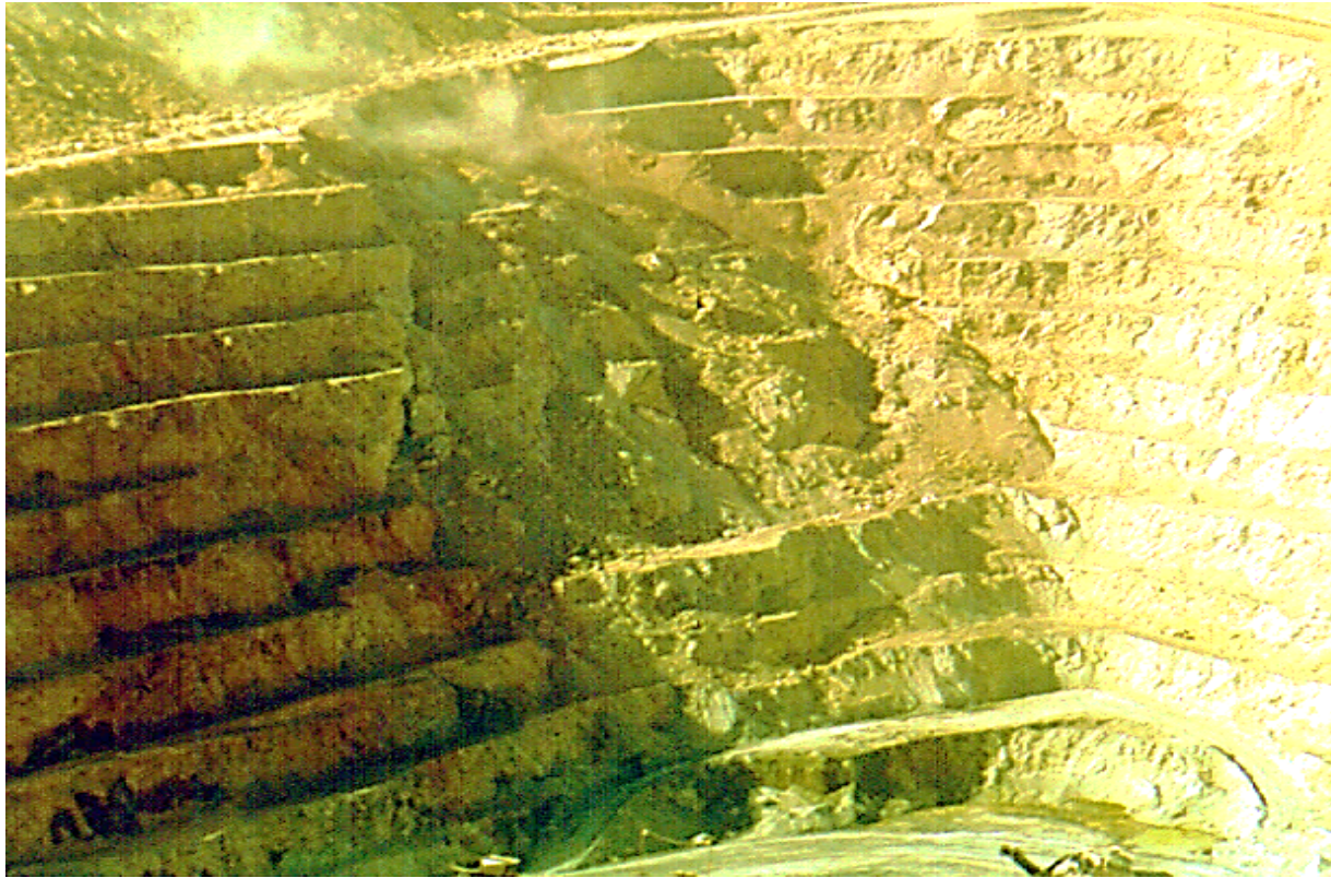
Figure 1: Slope failure in which some structural control by faults is evident at the top of the failure, but where the mechanisms involved in the low part of the failure are unclear.
