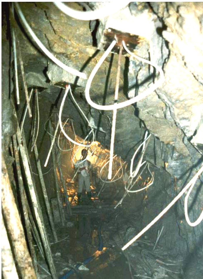
Figure 14: Untensioned grouted cables installed from the longitudinal working galleries to pre-reinforce the rock mass above the power cavern roof.
