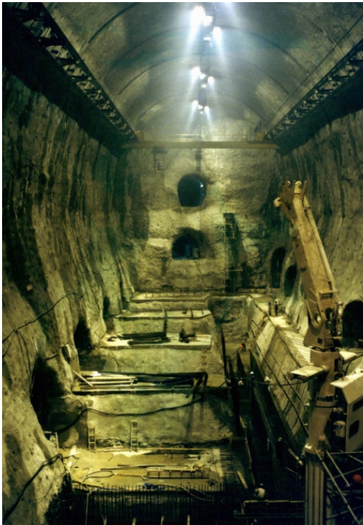
Figure 28: Crane beam anchored to the curved wall of the elliptical power cavern of the Singkarak hydroelectric project in Indonesia.
