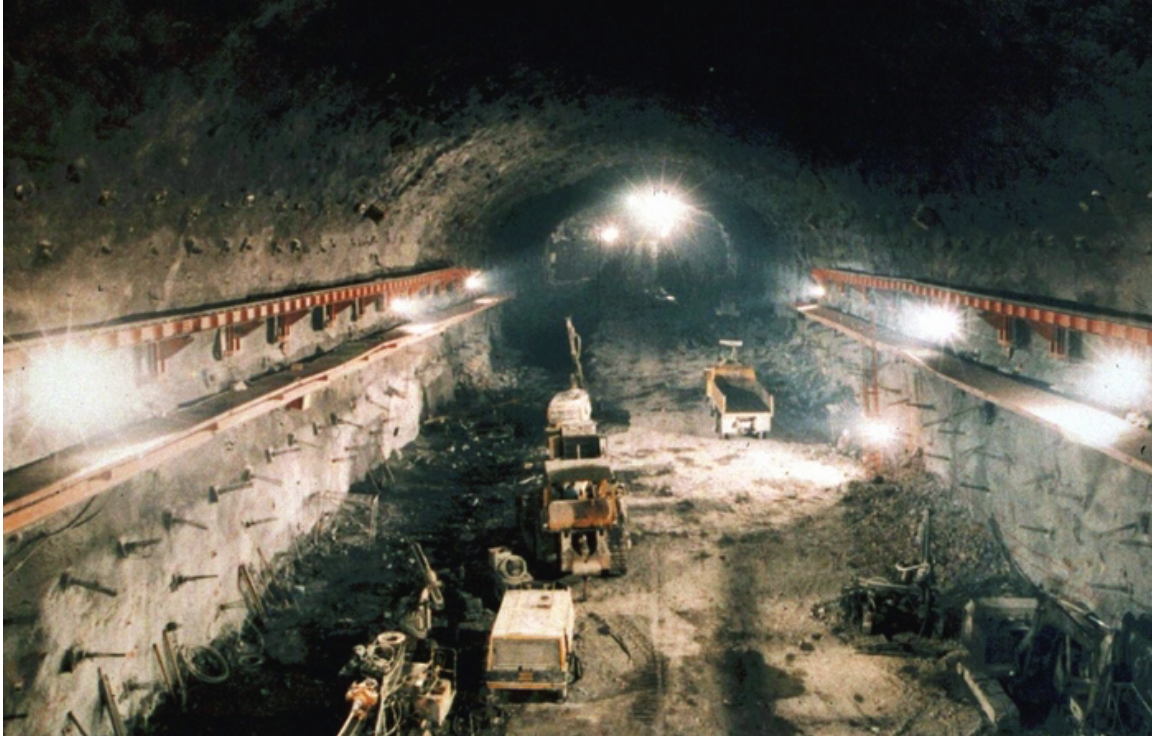
Figure 25: View of the Mingtan cavern from the platform of a temporary construction crane supported on rails bolted to the cavern walls.
