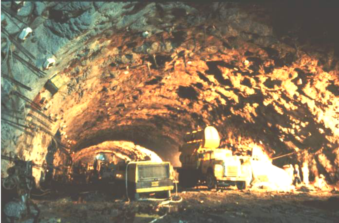
Figure 19: Completed excavation of the cavern arch.
