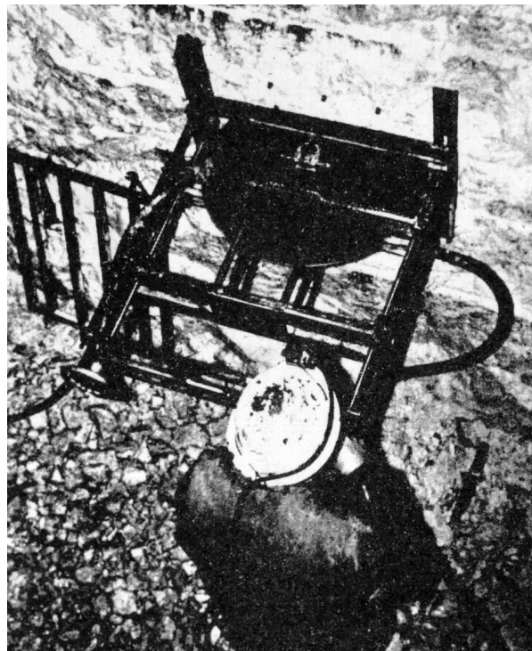
Figure 10. Flat jack test - cutting a slot with a circular saw. (Photograph by courtesy of S.E.I.I., Paris ).
