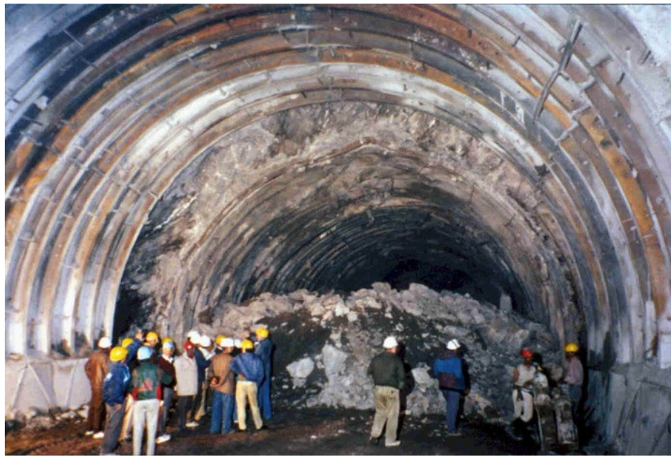
Fig. 10: Large convergence in the Nathpa Jhakri headrace tunnel top heading due to the influence of the Daj Khad shear zone.
