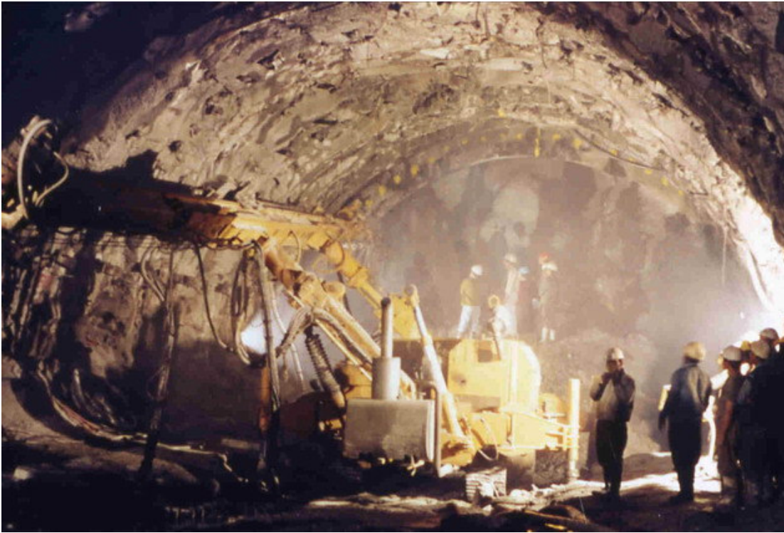
Fig. 16: Installation of 12 m long grouted pipe forepoles to form a protective reinforced rock umbrella under which excavation of the top heading can proceed.
