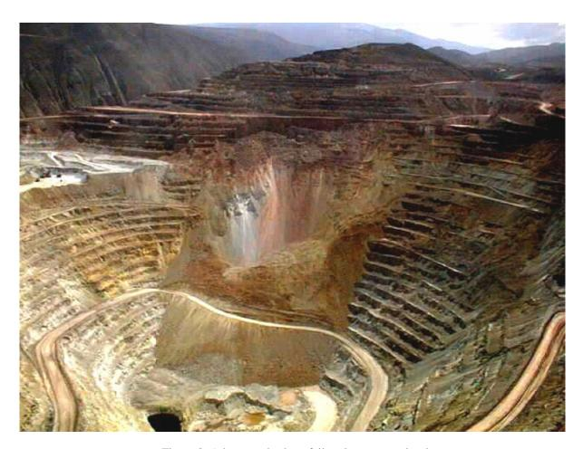
Figure 2: A large scale slope failure in an open pit mine.
