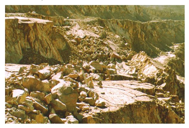
Figure 11: Large deformations in the West wall of the Chuquicamata Open Pit Mine in Chile.
