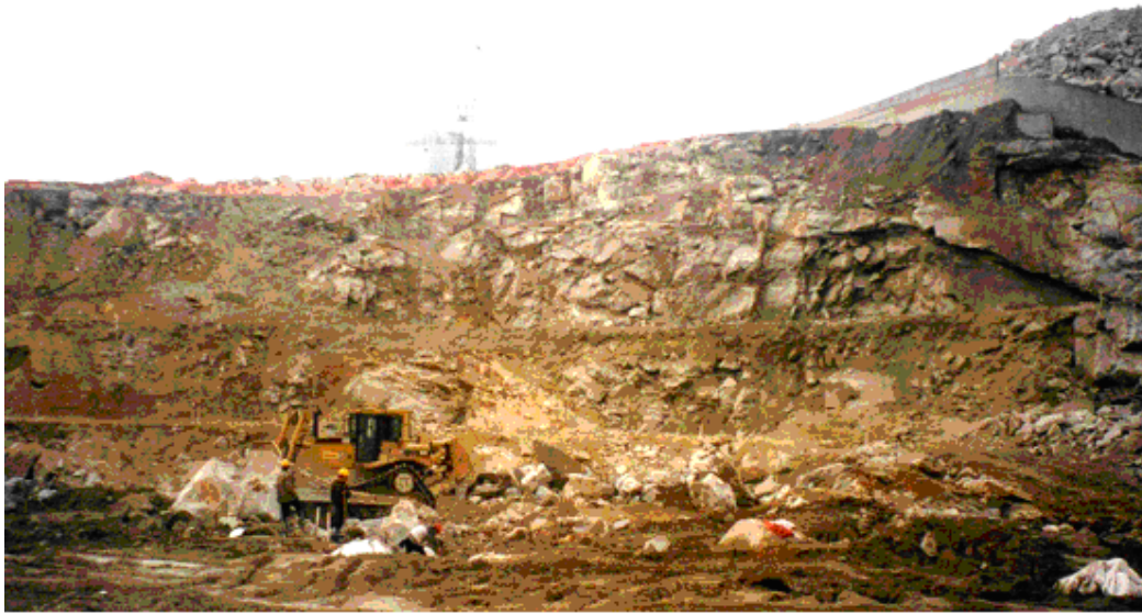
Figure 4: Appearance of Oporto granite in the face of an excavation for the new football stadium. Fracturing of the rock mass and heterogeneity of weathering is obvious
