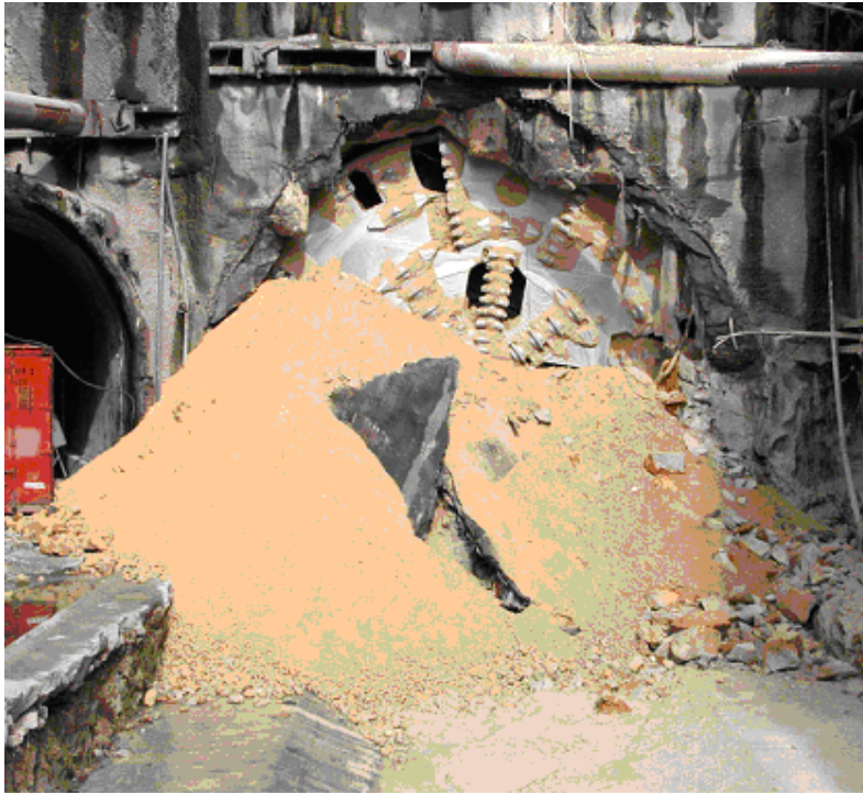
Figure 13: Final breakthrough of the TBM S-203 on the completion of the drive from Salgueiros to Trindade on Thursday 16 October 2003.
