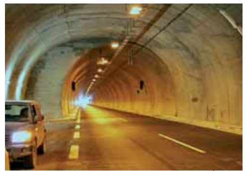
Above: a parking bay in a typical operating tunnel on the Egnatia highway
