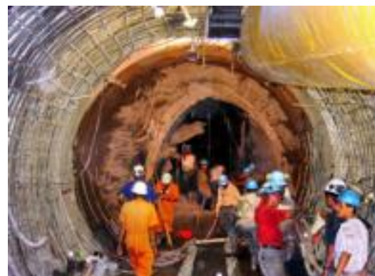
b. Rehabilitation of collapsed tunnel
