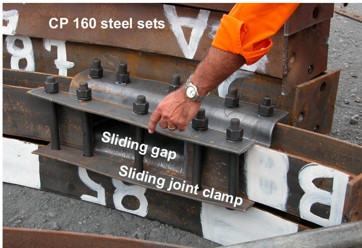
Figure 22: Details of one of the two sliding joints in the steel sets.
