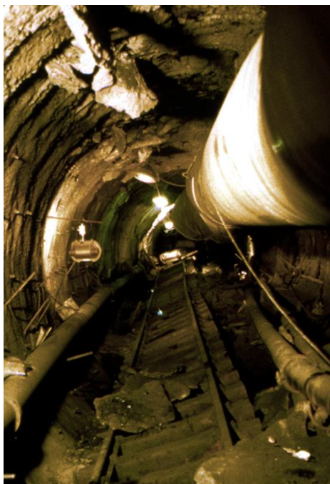
Figure 6: Floor heave about 100 m behind the Intake drive TBM in 1979 at a depth of 400 to 425 m below surface.
