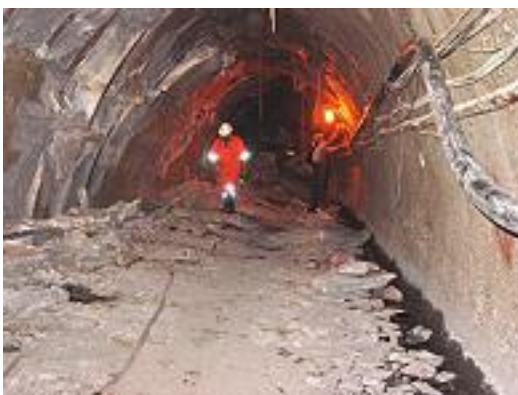
a. Damage to invert and arch
