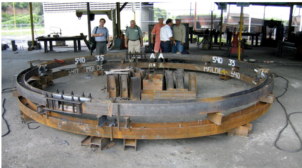
Figure 23: Assembled steel set with two sliding joints in the site workshop.
