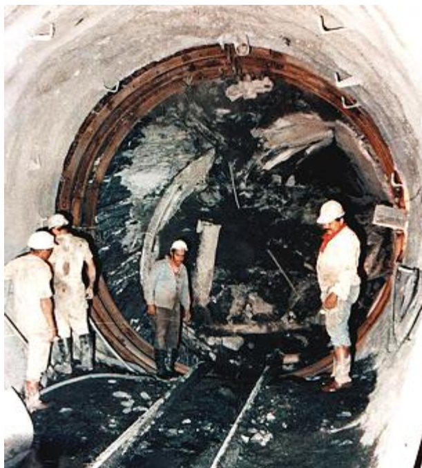
Figure 7: Excavation of the remains of the TBM in 1987 during the fourth contract.
