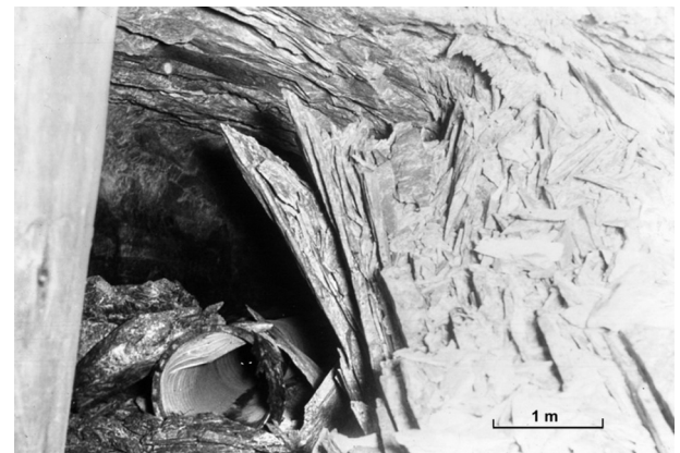
Fig. 25. Severe rockbursting in an access tunnel in a deep level gold mine in South Africa.
