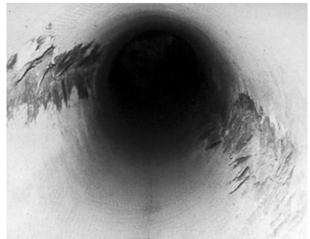
Fig. 24. Mild spalling in the sidewalls of a vertical raise bored shaft in an underground mine.
