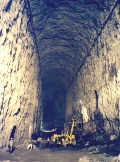
Figure 26: Partially completed 20 m span, 42.5 m high underground powerhouse cavern of the Nathpa Jhakri Hydroelectric Project in Himachel Pradesh, India. The cavern is approximately 300 m below the surface.
