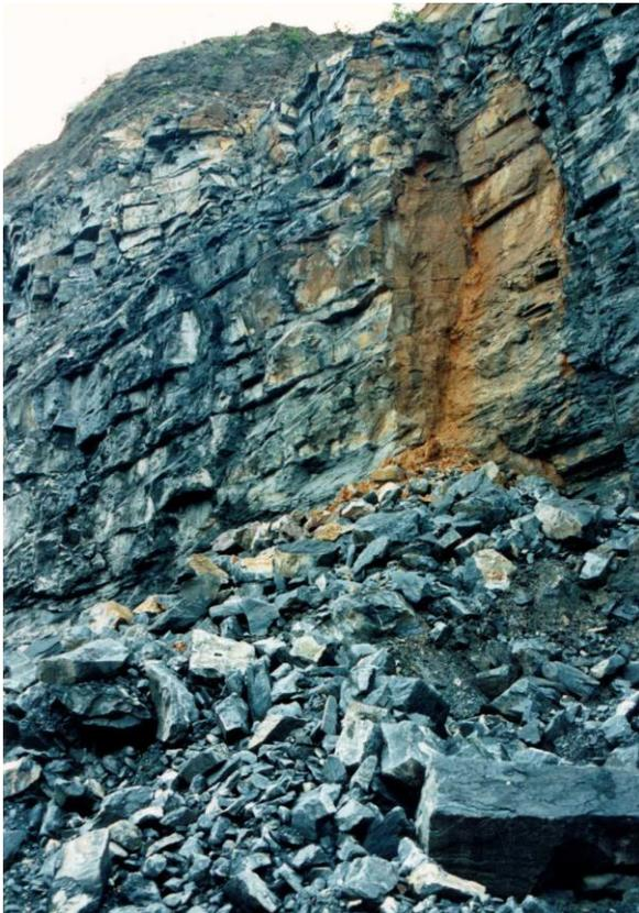
Figure 35: Structurally controlled failure in the face of a steep bench in a heavily jointed rock mass.
