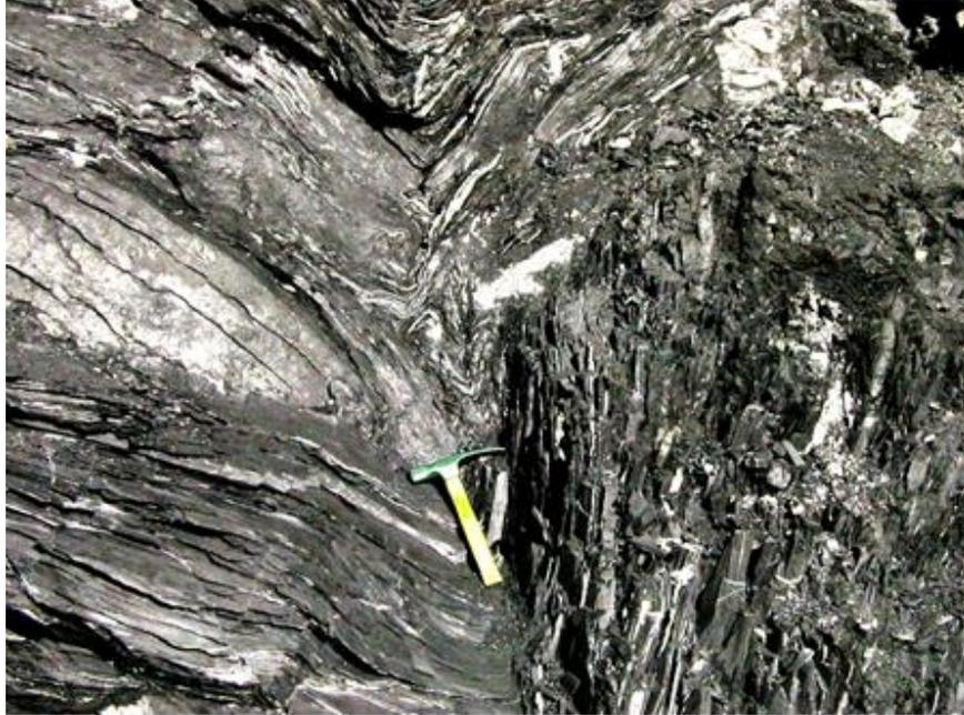
Figure 3: Yacambú-Quibor graphitic phyllite in the tunnel face.
