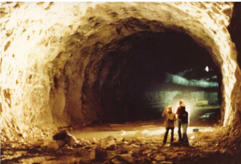
Figure 26: Top heading of the 12 m span, 18 m high tailrace tunnel for the Rio Grande Pumped Storage Project.
