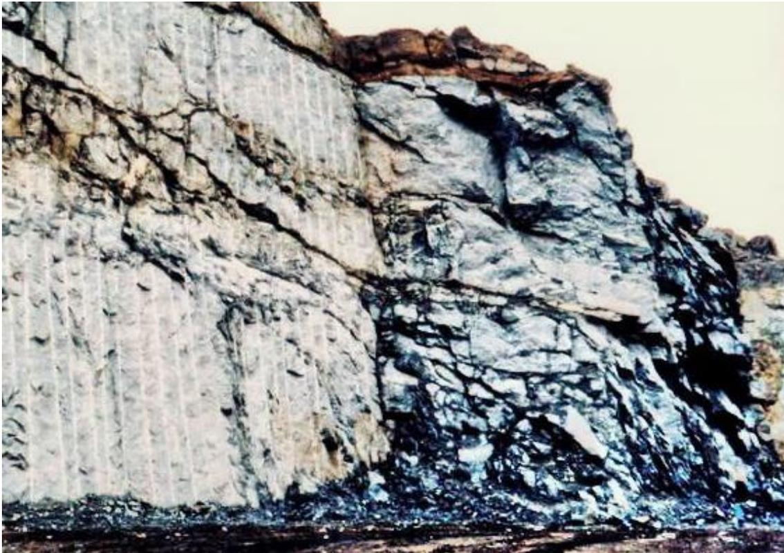
Figure 8: Comparison between the results achieved using controlled blasting (on the left) and normal bulk blasting for a surface excavation in gneiss.
