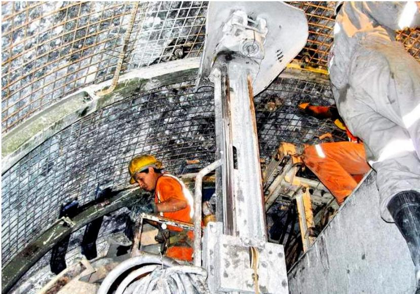
Figure 6: Wire mesh, used in conjunction with steel sets and/or rockbolts, is very effective for the support of blocky rock, particularly in tunnelling using a TBM, as shown in this figure. It also provides effective reinforcement for the shotcrete layer.
