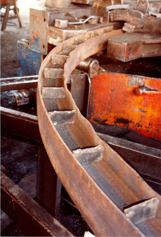
Figure 12: Buckling of an H section steel set being bent to a small radius. Temporary stiffeners have been tack welded into the section to minimise buckling but a considerable amount of work is required to straighten the flanges after these stiffeners have been removed.
