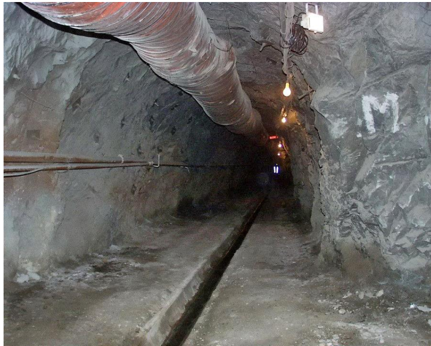
Figure 10: Appearance of the drainage tunnel in fair quality granodiorite in which no permanent support was required. Spot bolts and shotcrete were installed for safety in jointed areas. The concrete lined drainage channel is shown in the centre of the tunnel floor.
