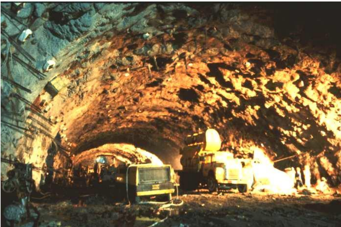
Figure 19: Completed excavation of the cavern arch.
