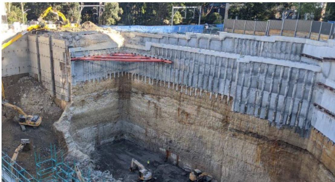
**Figure 5: Excavation support along Sydney Trains (west) boundary**
