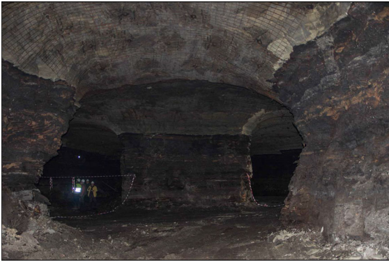
Fig. 19 View of the underground exploitation after the completion of the stoping activity
