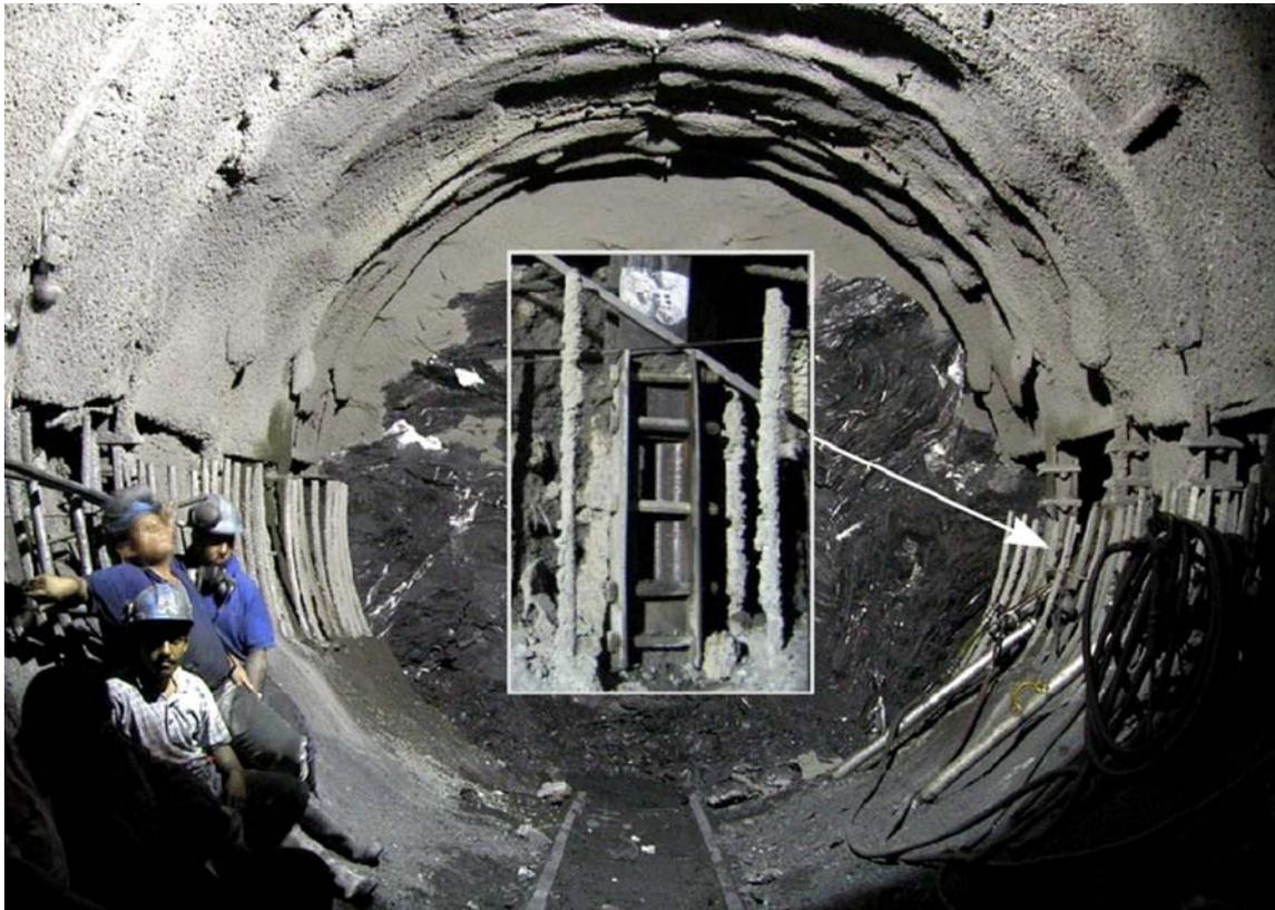
Figure 9: Installation of a circular lining in heavily stressed rock. The inset shows the sliding gap and the shotcrete window over this gap. Reinforcement for the second layer of shotcrete is visible in this shotcrete gap.
