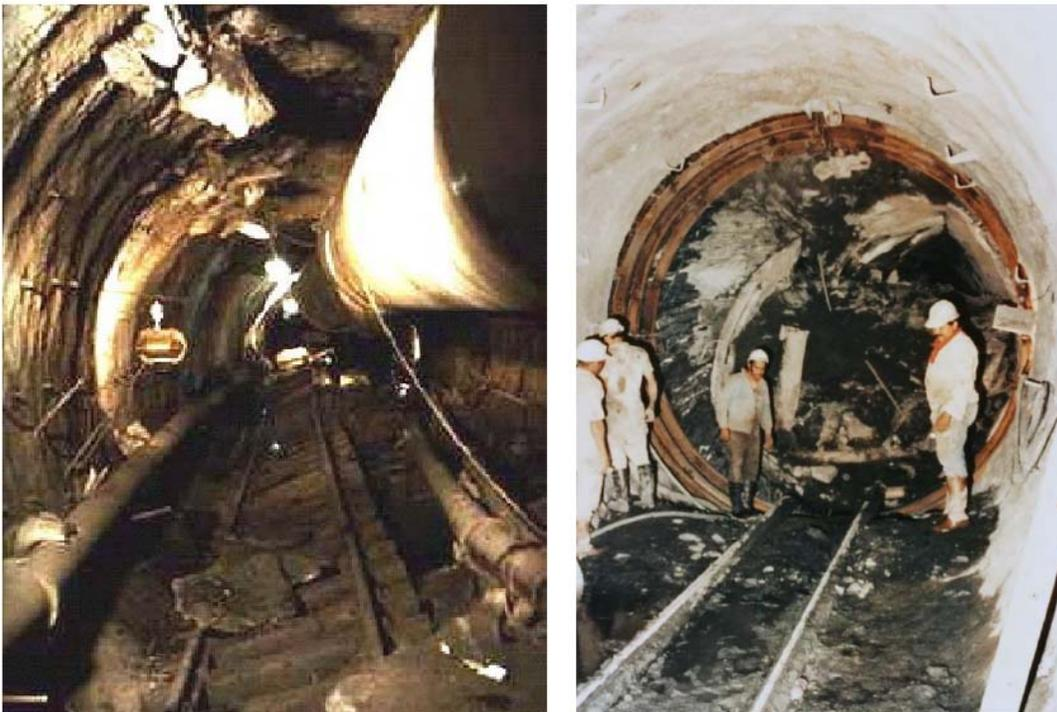
Figure 4. Left: Floor heave about 100 m behind the Intake drive TBM in 1979 at a depth of 400 to 425 m below surface. Right: Excavation of the remains of the TBM in 1987 during the fourth contract.
