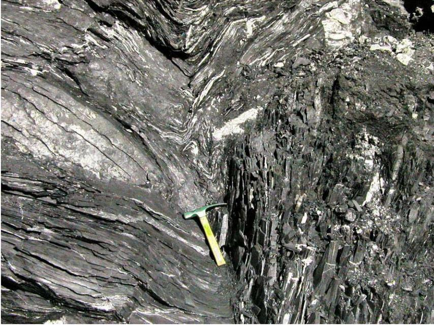
Figure 3. Tectonically deformed graphitic phyllite at the tunnel face.
