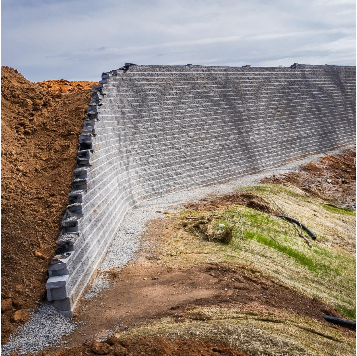
Figure 1.1: Illustration of a segmental block retaining wall
