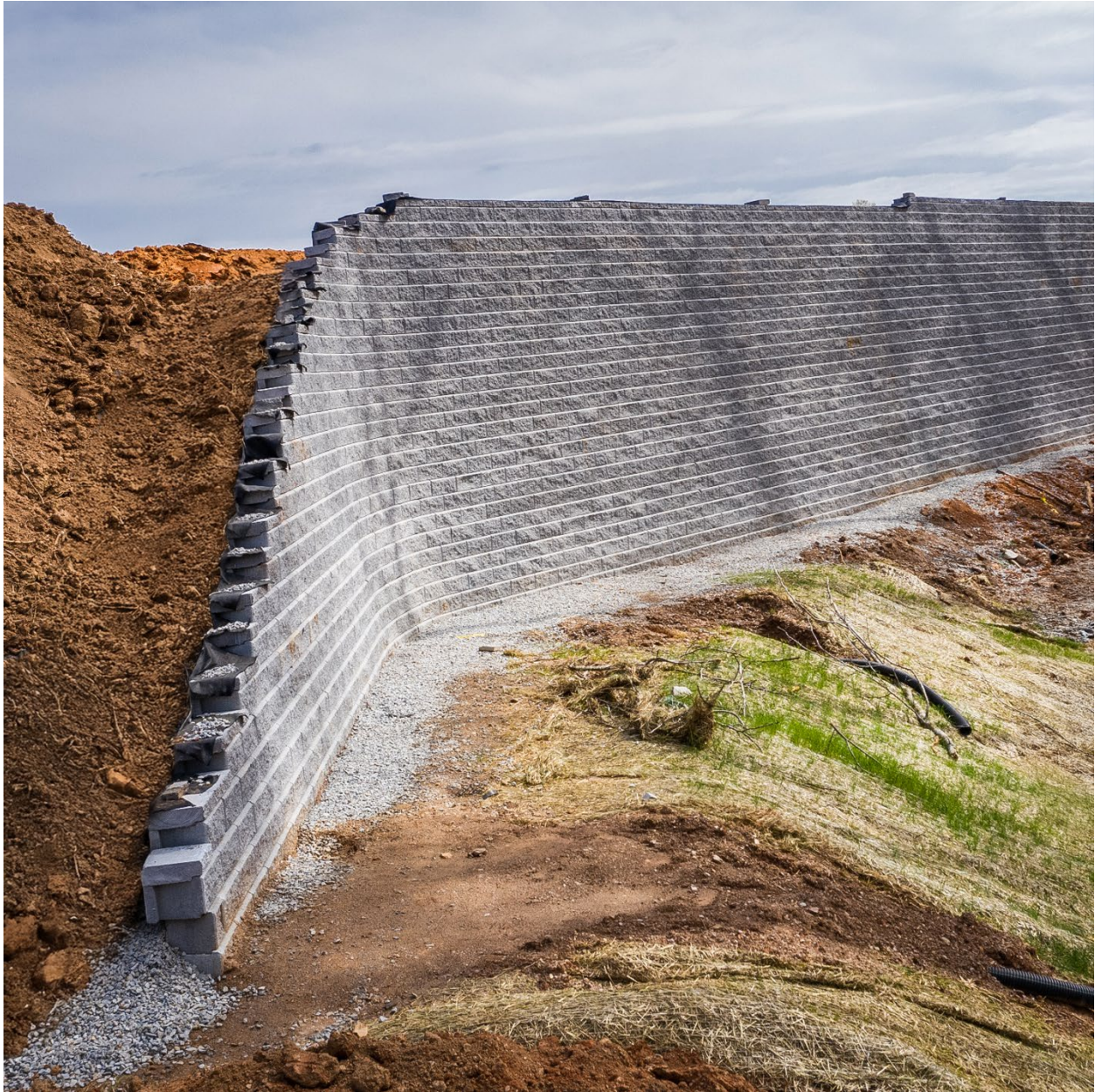
Figure 1.1: Illustration of a segmental block retaining wall
