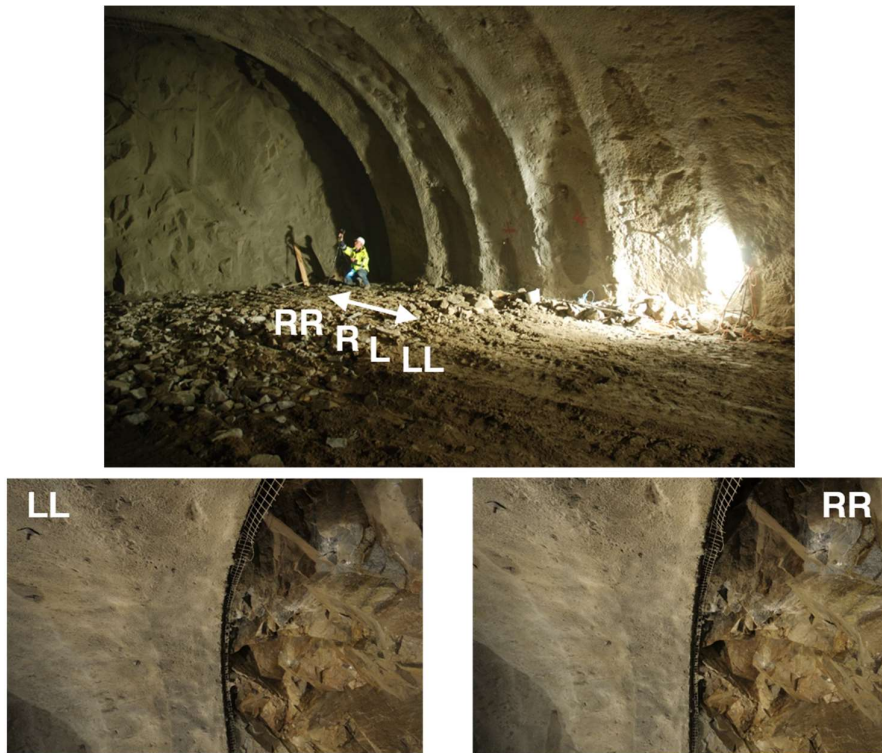
Figure 21: Example of imaging the left springline
