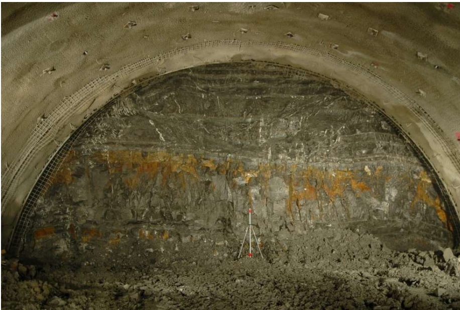
Figure 36: Range Pole installed in front of a tunnel face. The Range Pole should be located leading to minimum occlusion of the face behind. It can be placed in the middle , at the sides or at any position visible in both images but not too close to the camera locations.
