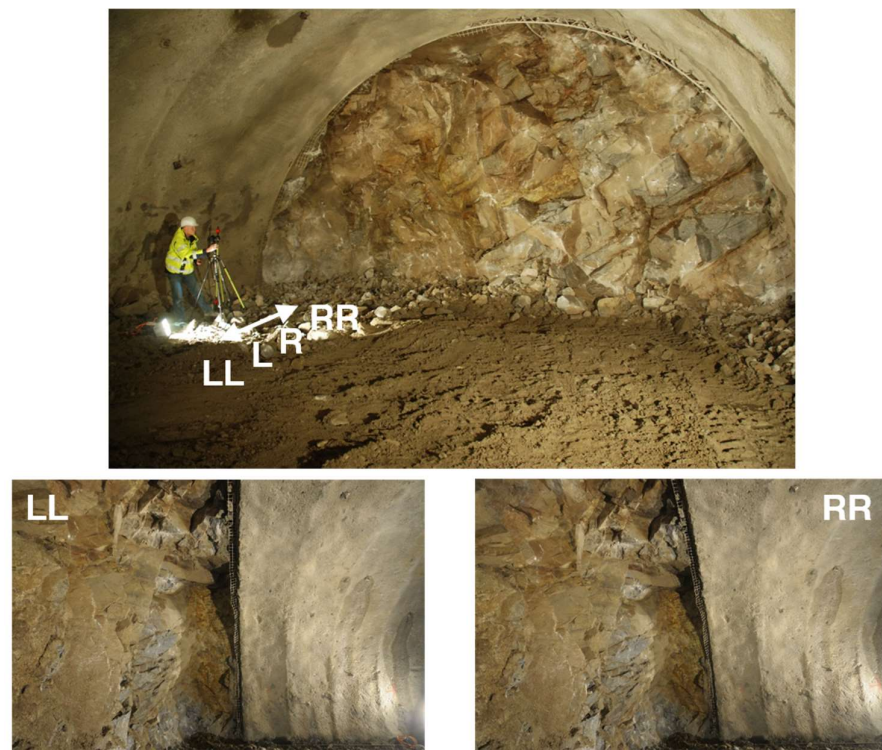
Figure 22: Example of imaging the right springwall
