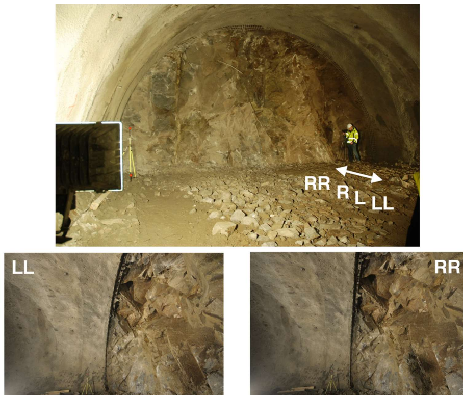
Figure 20: Example of imaging the left sidewall
